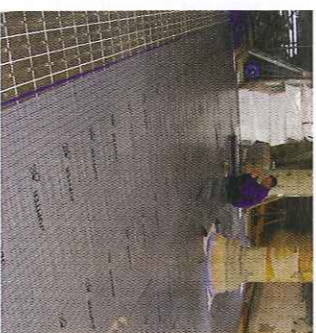
EPS Edge Zone panels were covered with a protective membrane (above), over which the heating system and Screed Replacement Tiles were laid. The final floor finish (right).
