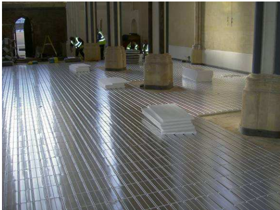
JUPITER IDEAL EPS panels being installed. Pipe centres are 125mm.
