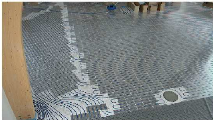
Jupiter IDEAL EPS system installed at Mary Immaculate & St Gregory RC church in Barnet
